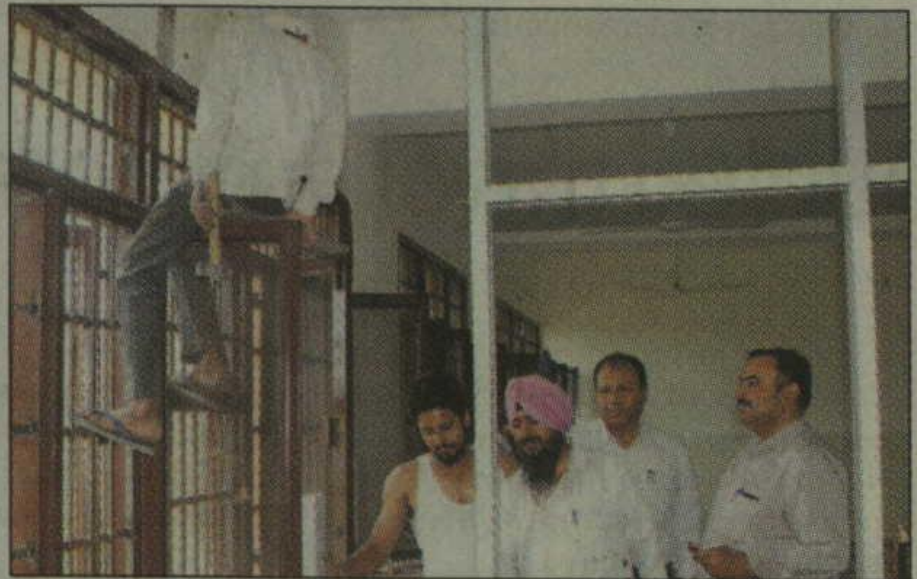
Work in progress at IIM Amritsar's temporary campus in Amritsar.
